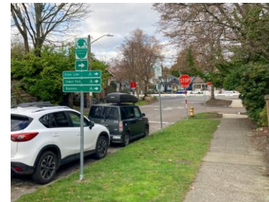
The U-District Neighborhood Greenway, which has been extended at the 12th Ave NE and NE Ravenna Blvd "triangle" with new wayfinding signs, updated sidewalks and curb ramps, speed humps, and new stop signs to make travel safer and more predictable.
