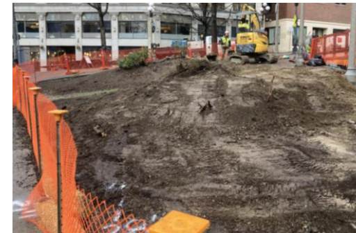
Construction underway on Fortson Square.
