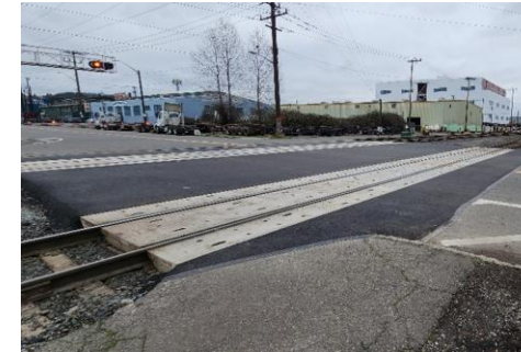
Repaired crossing surface at S Hanford St
