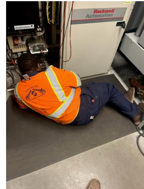
Performing electrical preventative maintenance on the Ballard Bridge.
