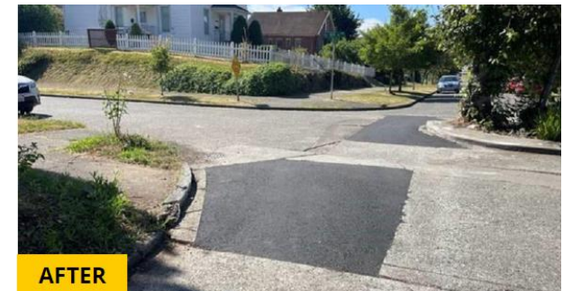
Before and after a repaving project on 16th Ave S. We removed damaged concrete panels and patched with full-depth asphalt.
