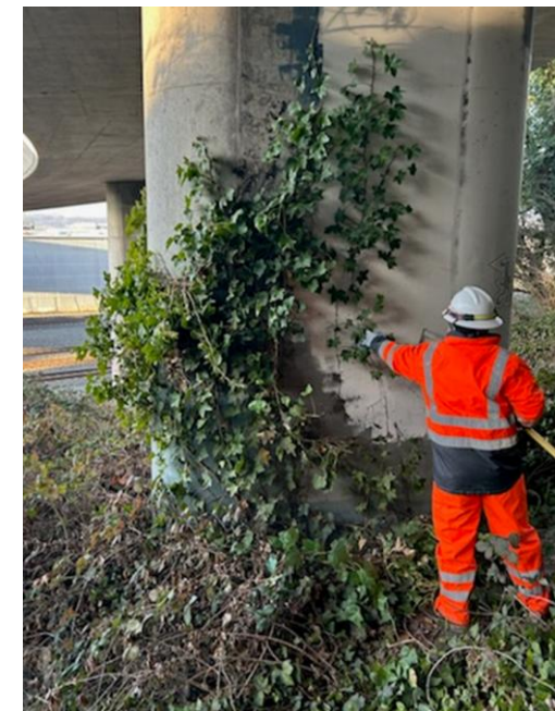
Bridge cleaning on a bridge on S Lucile St.
