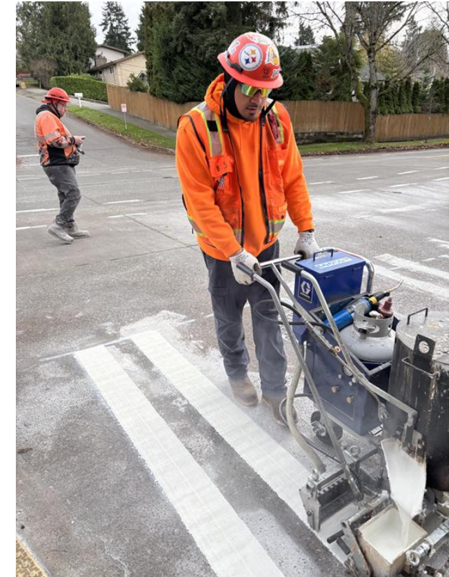
SDOT crews remarking sidewalks on SW Myrtle St and 16 th Ave SW.
